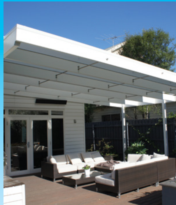
Posts and beams
