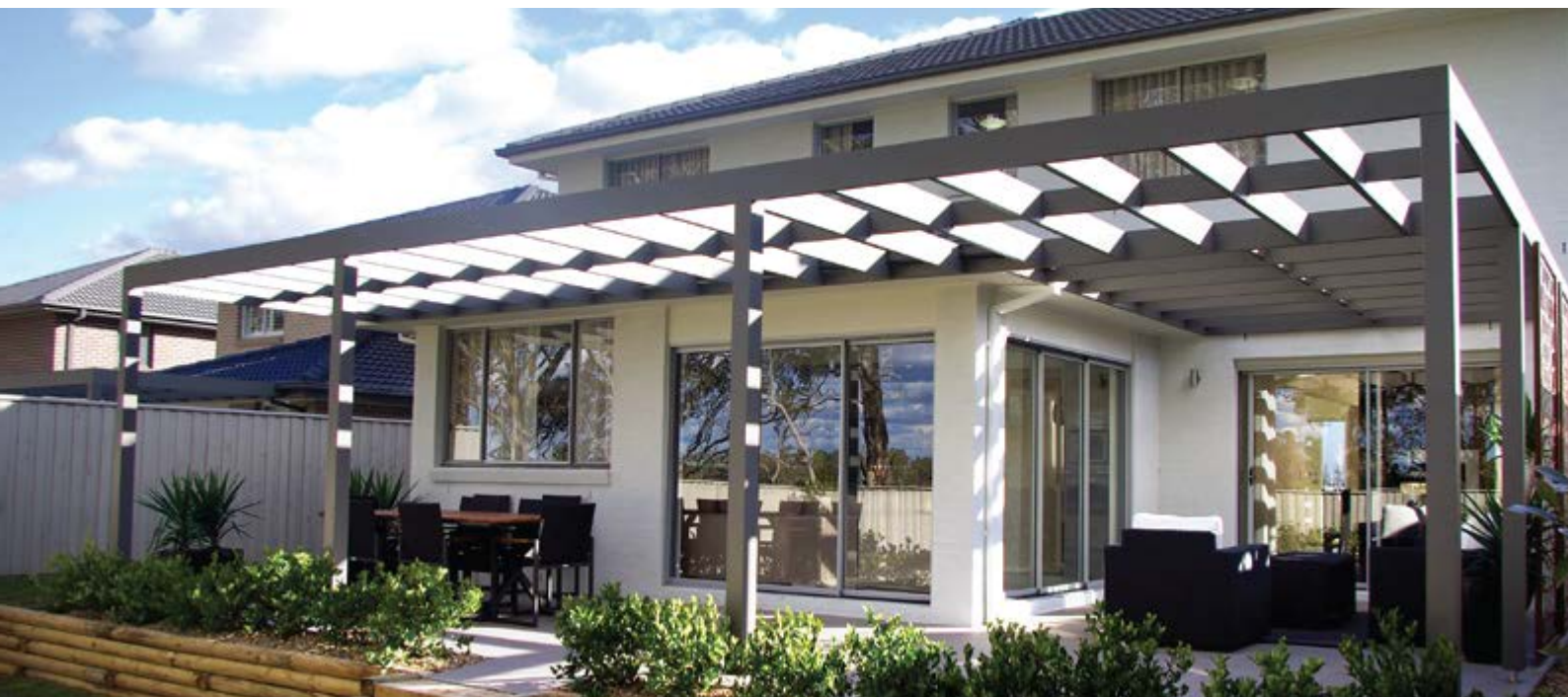
Posts, beams and rafters
