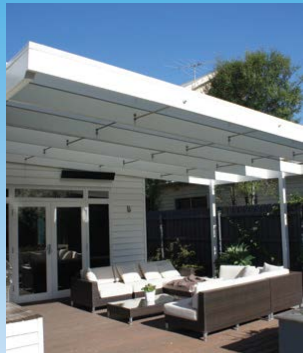
Posts and beams
