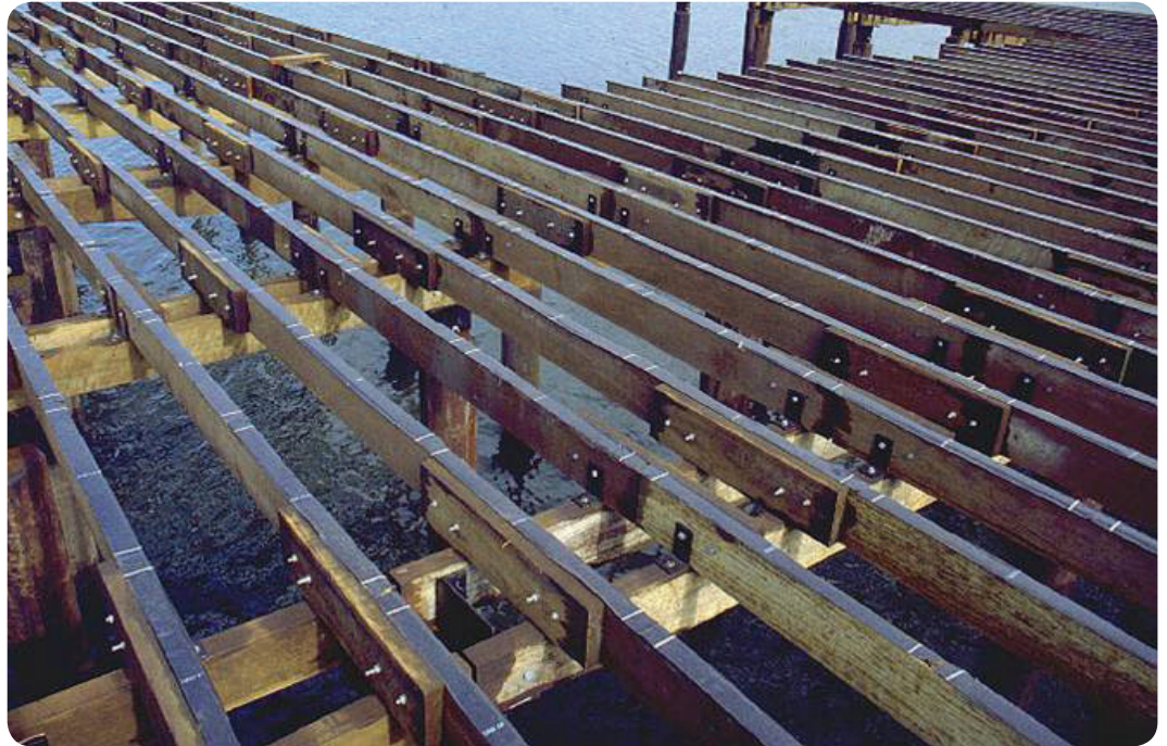
Bituminous DPC fixed to top of deck joists.
