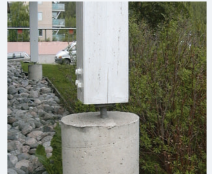
A well-ventilated, free-draining post support.
