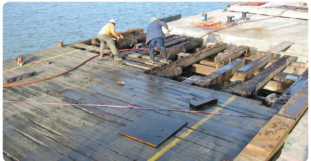
Wharf timbers to be recycled and re-used after approximately 60 years in-service.
