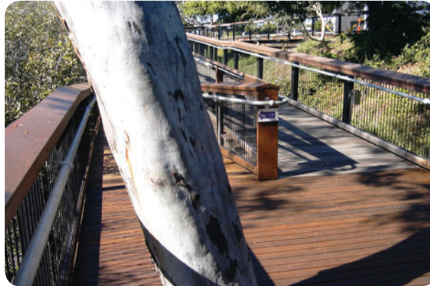
Public boardwalk in process of maintenance with decking oil.
