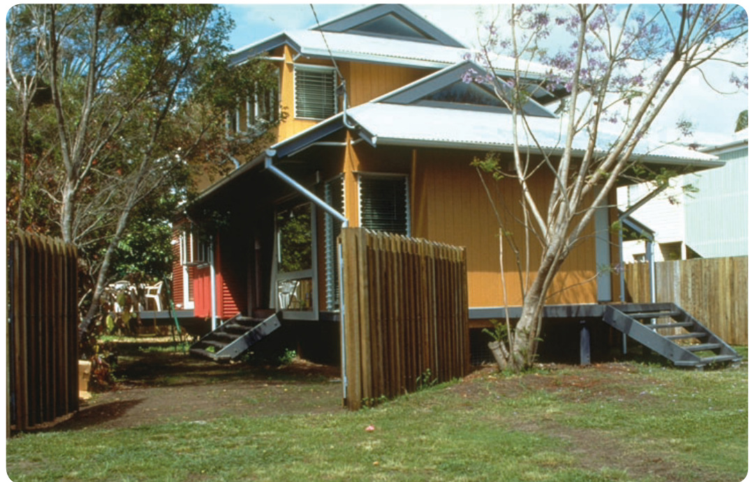
Large overhangs provide good protection.
