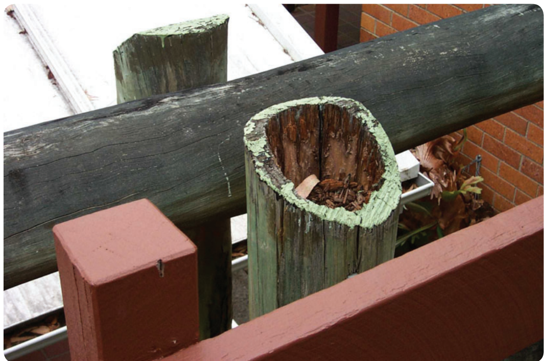
CCA treated sapwood outperforming durability class 2 heartwood
