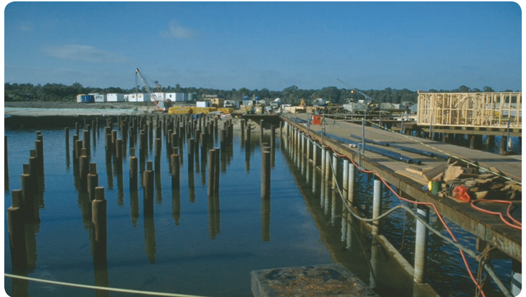
Double treated marine piles at Couran Cove, Queensland.
